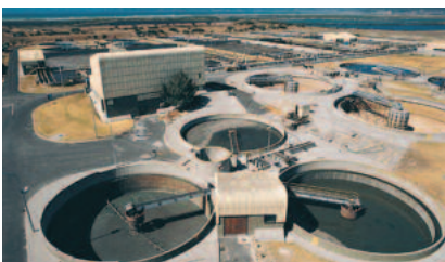
Flexible and reliable communication is a key issue in many application regardless of scale and size.
