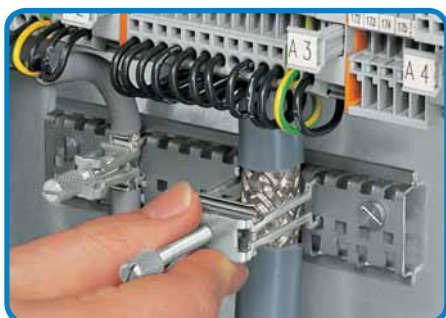
Addition of a shield (screen) clamping saddle.
