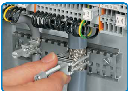
Addition of a shield (screen) clamping saddle.
