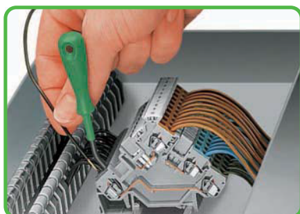
The blade dimensions of the above-listed operating tool (DIN 5264) are ideal for easy operation of 280 Series front-entry sensor and actuator terminal blocks.
