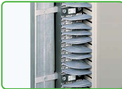
Matrix patchboards in a frame.
