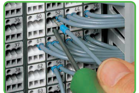
Terminating ferruled conductors.
