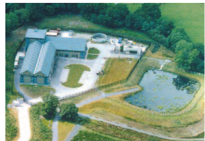
Example of remote pumping station.
