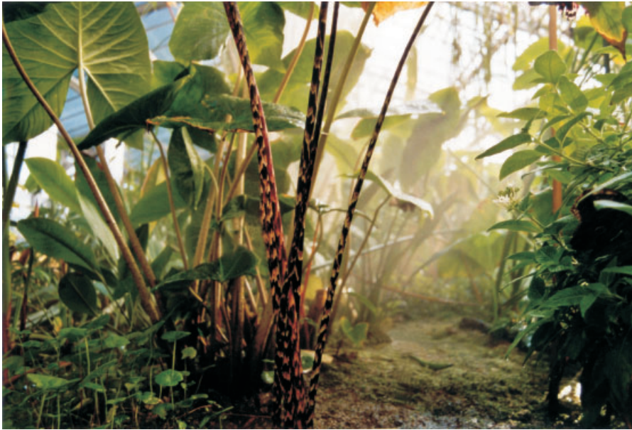
Alpha controllers can automate many tasks, for example greenhouse watering, heating and vent control
